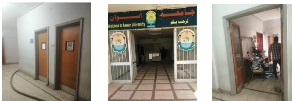
Fig. 14 The interior doors' widths are 80–90 cm (2020)
