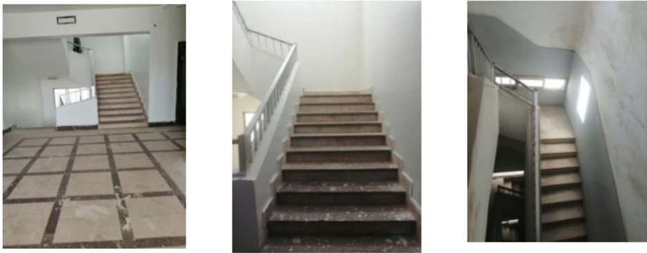
Fig. 11 The main stair is 1.7 m in width, while the emergency stair is 1 m in width (2020)
