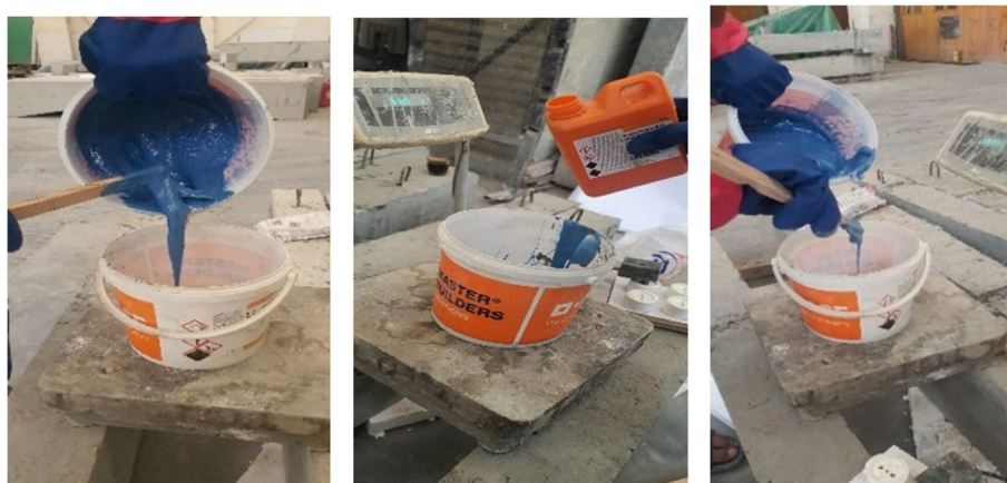
Fig. 3 Applying epoxy resin
