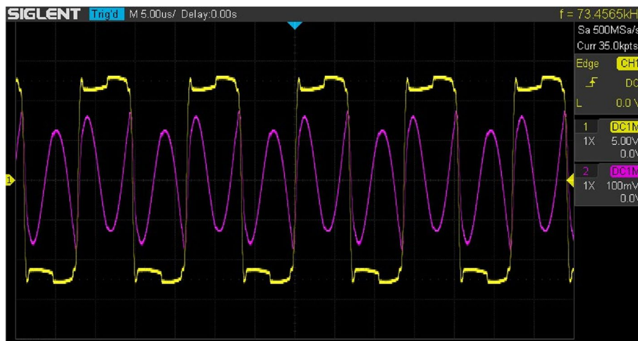
Fig. 7 Inverter voltage (yellow) and current (pink) of a parallel resonant induction heater with low matching inductor
