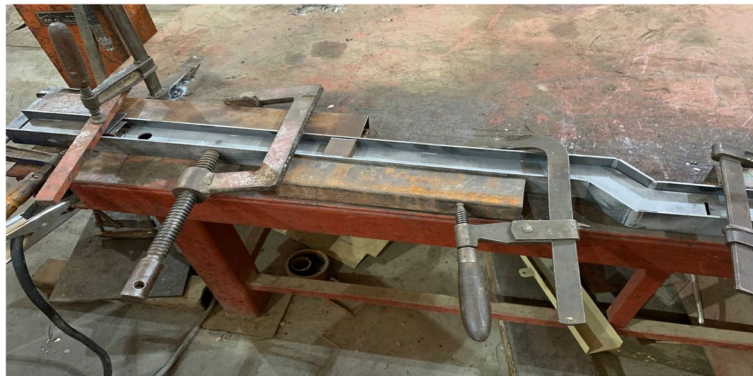
Fig. 11 Assembling the main longitudinal beam by a fixture for welding
