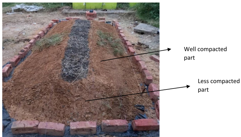
Fig. 9 Grass placed over a length on both sides of compacted embankment
