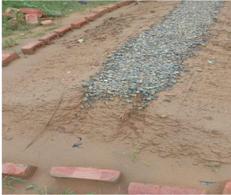
Fig. 16 Showing two newly formed gullies on lateral side
