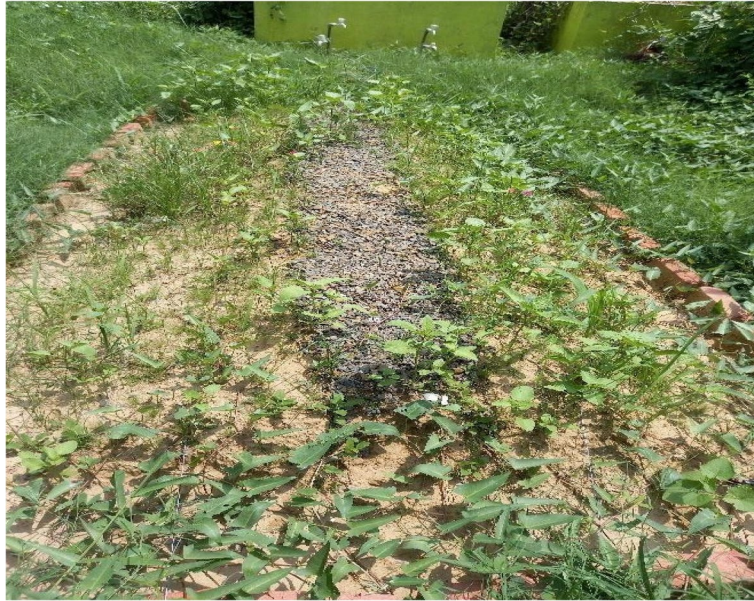
Fig. 18 Shows growth of vegetation on embankment
