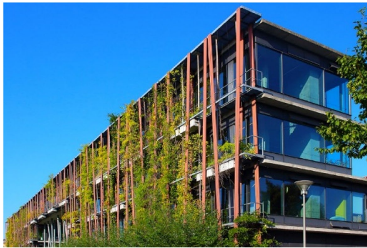
Fig. 3 The facades of the Institute of Physics at Humboldt University, Berlin, Germany [10]. Its facades include rainwater management and energy savings with natural air conditioning through plant walls
