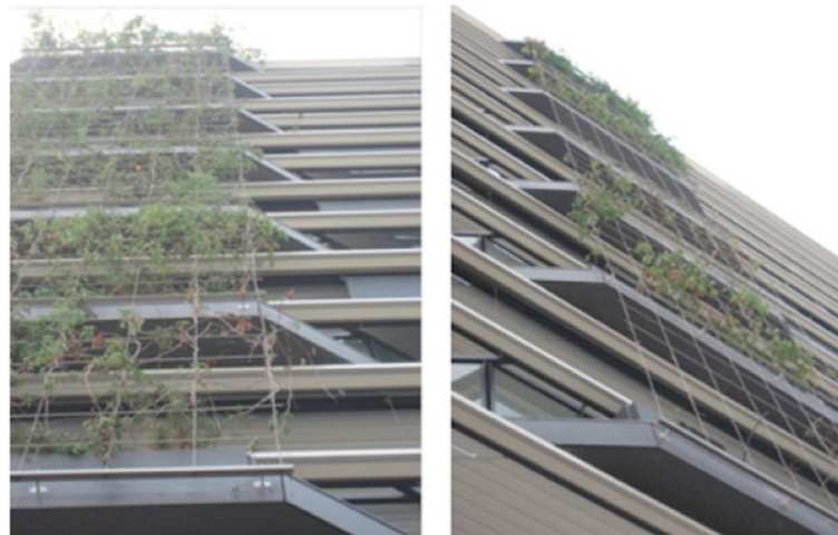
Fig. 2 The system of cables and wiring for the climbing plant [14]. The two systems use high-tensile steel cables and related equipment. The wiring system is more flexible than the cable system and allows for greater design space. It may be adjusted in both vertical and horizontal dimensions to accommodate an endless number of different sizes and styles
